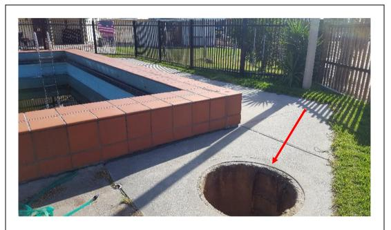
**Image 9.** Pit at NE corner, 1.65m to water level. Expected purpose is ground water pump out.
